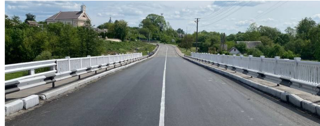
Bridges across the Sluch River in Zhytomyr Region
