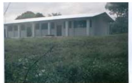
FRONT VIEW OF THREE CLASSROOM BUILDING OF THE K.K. GONAH PUBLIC SCHOOL, NEWLY RENOVATED.
